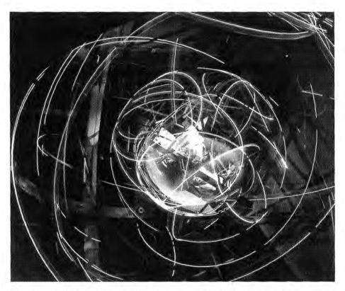
The epitome of human and machine interfaces, this device was formally known as the MASTIF, or Multiple Axis Space Test Inertia Facility, and was located in the Altitude Wind Tunnel in 1959. It was built at Lewis Research Center, now John H. Glenn Research Center, in Cleveland, Ohio, and was designed to train astronauts to regain control of a tumbling spacecraft. (NASA photo no. C1959-52233)
