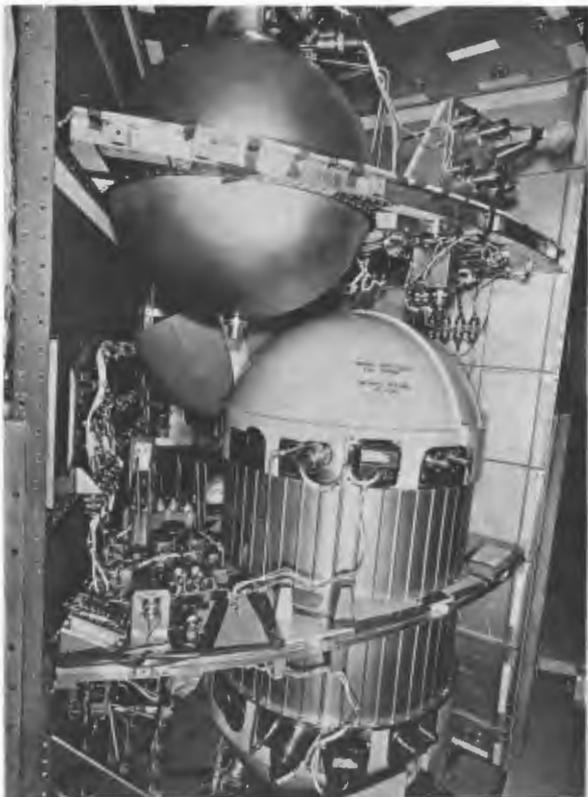
Beech Aircraft's cryogenic gas storage system—developed under contract let in 1964—supplied oxygen to the *Apollo 13* command module's environmental system in 1970 and hydrogen and oxygen to fuel cells for electrical power and drinking water. The system was in the *Apollo 13* service module. At upper left was one of two oxygen tanks. At lower right was a cylindrical housing jacket, rounded on each end, that enclosed two cryogenic hydrogen tanks.
