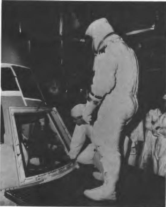
Astronaut Roger B. Chaffee prepares to enter Apollo spacecraft AS-204 in Kennedy Space Center's Manned Spacecraft Operations Building during October 1966 tests for the first manned Apollo mission. Phases of the mission—from countdown through liftoff, orbital insertion, and orbital exercises—were simulated in the altitude chamber.
