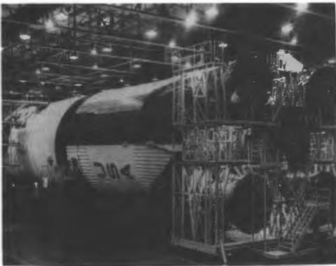
Five F-1 rocket engines, above, are installed in the massive first flight S-IC stage of the Saturn V launch vehicle at NASA's Michoud Operations plant in New Orleans. At right, an F-1 engine is tested in the NASA High Thrust Test Area, Edwards, California. The rockets were developed under Marshall Space Flight Center direction by Rocketdyne Division of North American. Rocketdyne photos.
