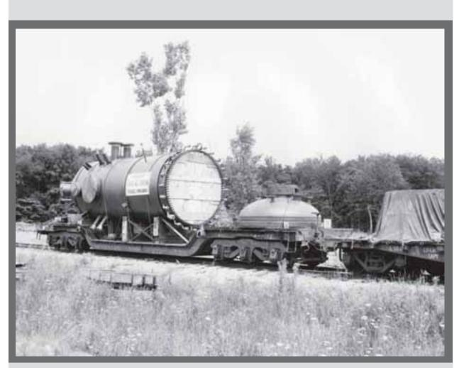
Image 45: The pressure tank was shipped to Plum Brook via railway, and transported to the reactor facility on a flatbed truck. The tank was then rolled to a crane, which lifted it into place at the center of the unfinished quadrant area. Several pipes jutted out from the tank. These "test holes" would be used to transport experiments to the reactor core for radiation during its operating cycles. (c. 1959) (NASA C-2003-833)
