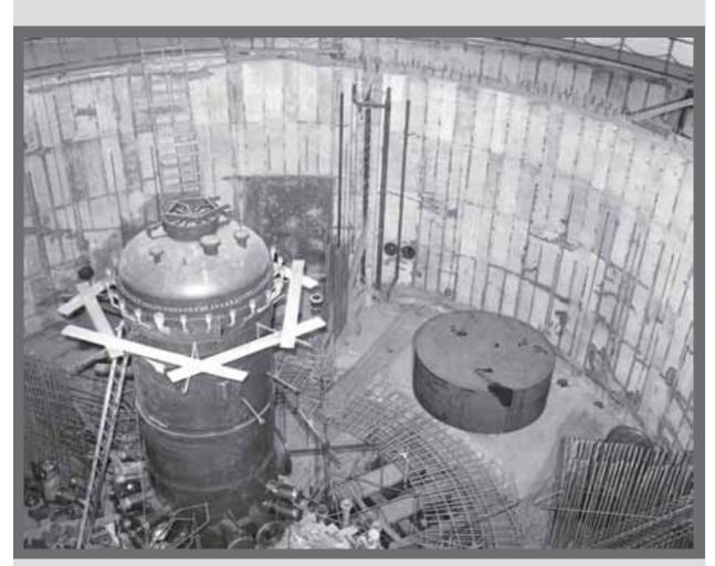
Image 49: The pressure tank in place inside the containment vessel. (NASA C-2003-836)
