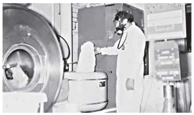
Image 82: A Plum Brook technician wearing protective clothing and a mask washes contaminated clothing. The clothing was worn again after it was decontaminated and laundered. The wash water had to be treated as radioactive waste. (2001) (NASA C-2003-841)
