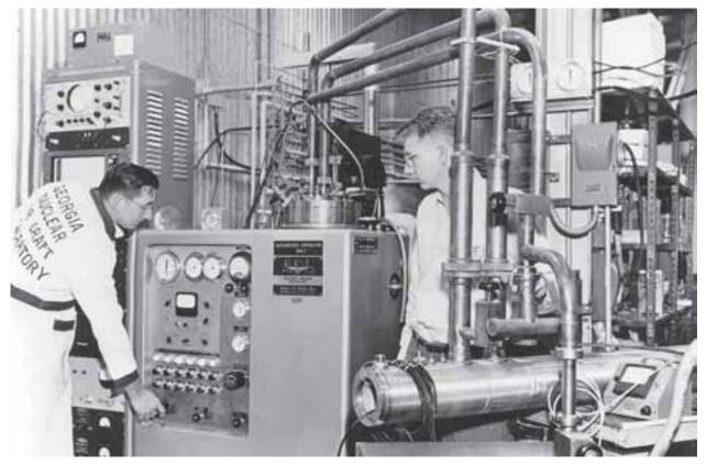
Image 97: Lockheed-Martin engineers make adjustments to the cryostat refrigeration machine that was being prepared for use in the Plum Brook Reactor Facility. The machine was used to test metals for their cryogenic resistant qualities. (January 1962) (Cleveland Public Library Photograph Collection, Ohio, Sandusky, Industry, NASA, Plum Brook Station)
