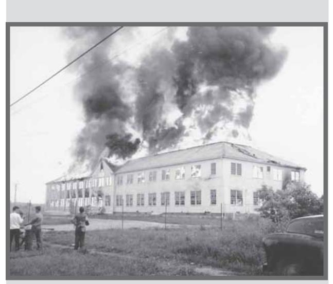
Image 40: Controlled fire to demolish unwanted Ordnance Works structure. Upon taking possession of Plum Brook, the NACA inventoried all the Ordnance Works structures and decided to retain forty-one of them, demolishing over 600 other buildings. In addition, three TNT areas and underground waste disposal lines had to be destroyed and decontaminated. (NASA C-2003-829)
