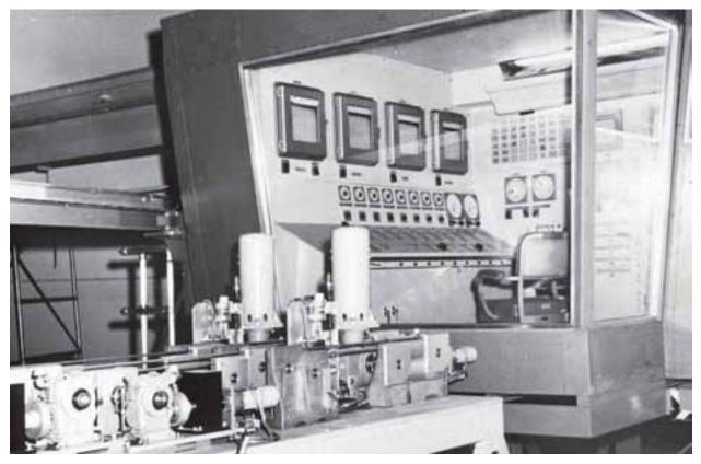
Image 71: The control room for the Mock-Up Reactor was perched directly above its core. The large windows allowed the operators to view the controls and monitors, as well as the activity in the core below. (NASA PS63–0008)
