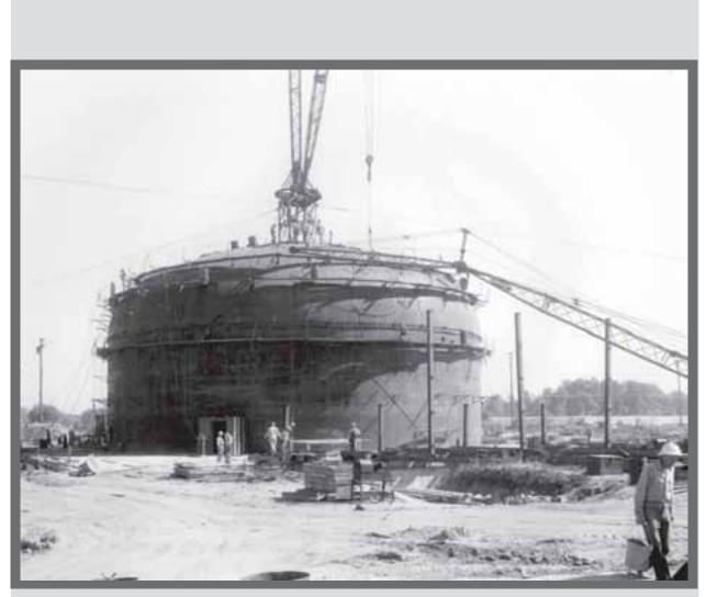
Image 43: Exterior of the containment vessel during construction. (NASA C-2003-831)
