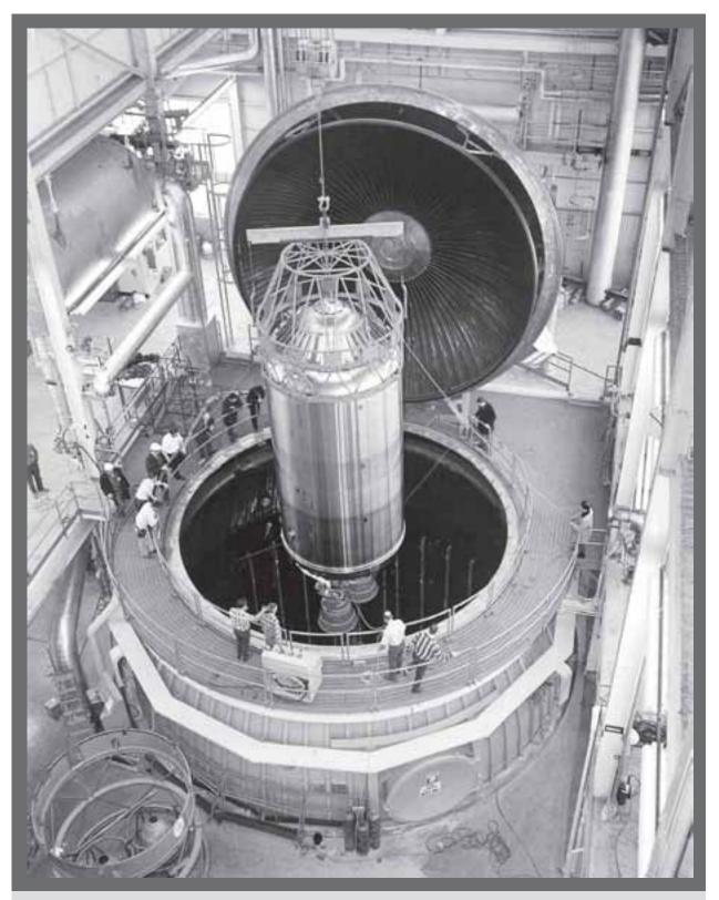
Image 111: The Spacecraft Propulsion Research Facility (B-2) was capable of testing space vehicles, and especially upper stage rockets like the Centaur, in a simulated space environment. The large vacuum test chamber could accommodate vehicles as large as 22 feet in diameter and 50 feet in length. The facility stood 74 feet high and extended 176 feet below ground. (NASA C-1999–00305)
