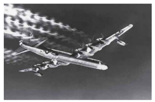
Image 26: The aircraft in these photos, a B-36 bomber converted to run a nonpropulsive test reactor during flight, flew fortyseven times between 1955 and 1957 over Texas and New Mexico. A nuclear-powered airplane was never flown. Engineers were aware of the multiple problems associated with an atomic plane, but they remained excited about the long-term possibilities. (Department of Energy)
