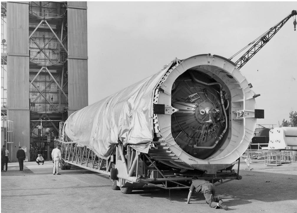
Image 209: Installation of the Atlas stage into E Stand (GRC-1963-P-01703).
