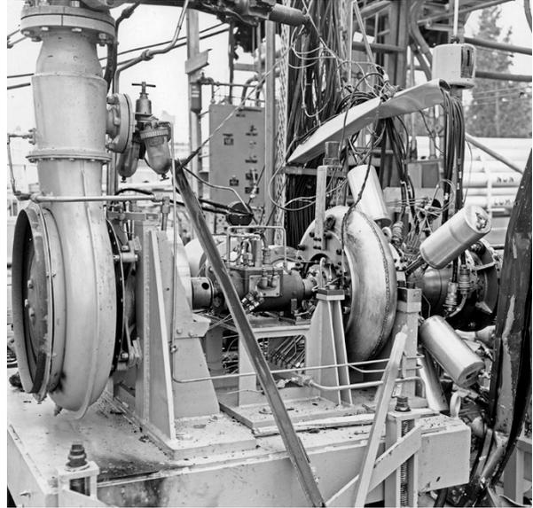
Image 216: Damaged equipment at the Pilot Plant (GRC-1964-P-01571).
