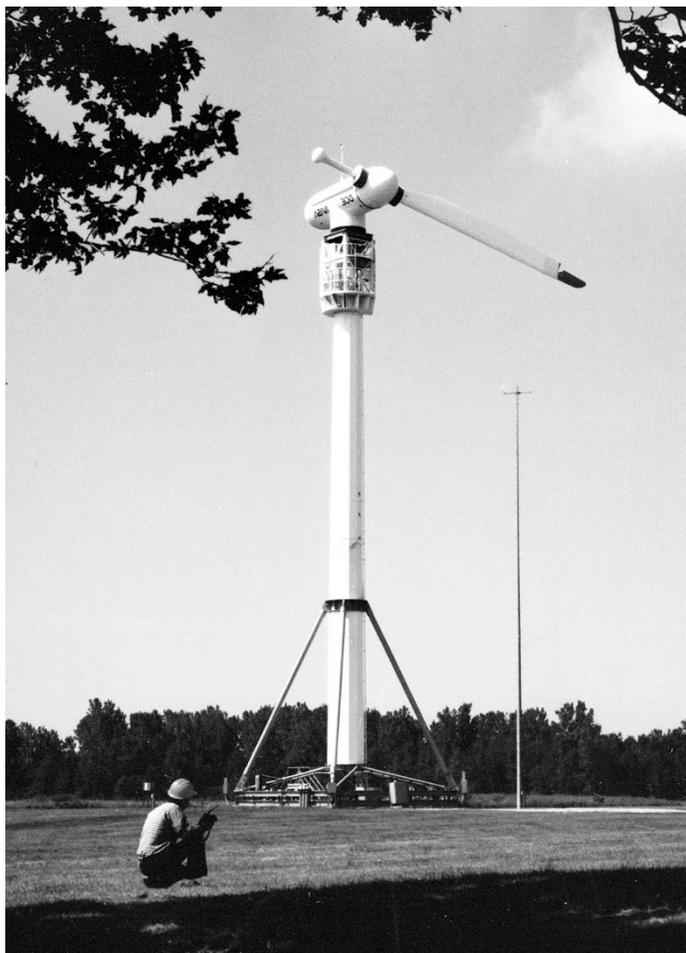
*Image 172: Single-bladed rotor. One of the most successful configurations used a lone blade with a counterweight on the other side. Despite concerns about the evenness and level of its power output, the single-bladed wind turbine generated over 200 kilowatts of power, twice the facility's original design capacity<sup>740</sup> (GRC-1985-C-05882).*
