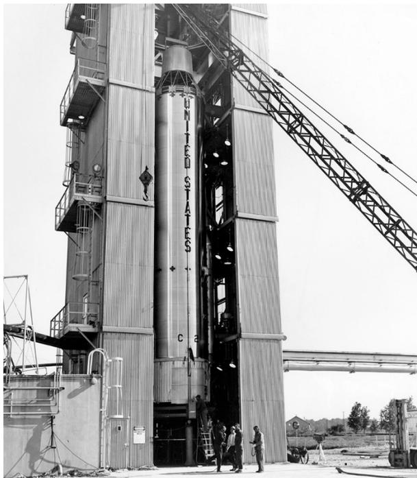
Image 207: Installation of the Atlas stage into E Stand (GRC-1963-P-01701).
