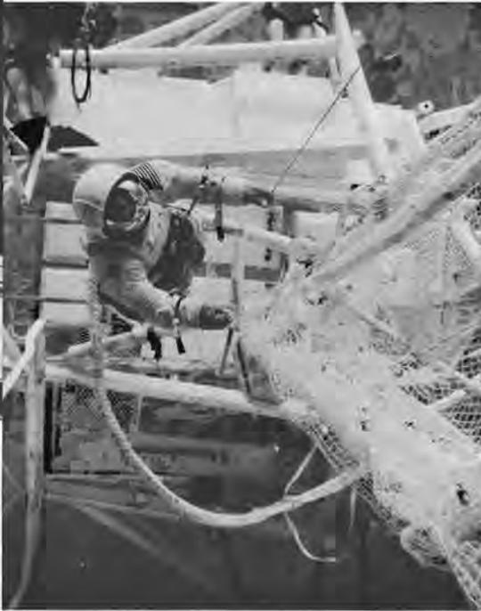
Two members of the Skylab 3 crew, Jack R. Lousma, left, and Owen K. Garriott, center, inspect a part of the twin-pole solar sail at MSFC (above). At right, Lousma practices erecting the solar sail over a portion of the Orbital Workshop mockup in the MSFC Neutral Buoyancy Tank. Nylon netting was used for this underwater training instead of the aluminized fabric the actual sail was made of.
