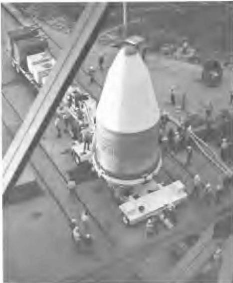
*Viking orbiter 1, top left, is mated to Viking lander 1 at Kennedy Space Center on 8 March 1975. Above, technicians lower the launch shroud over the spacecraft on 27 March. At left, the shrouded orbiter and lander move toward 31 March mating with the Titan III launch vehicle, for more tests.*
