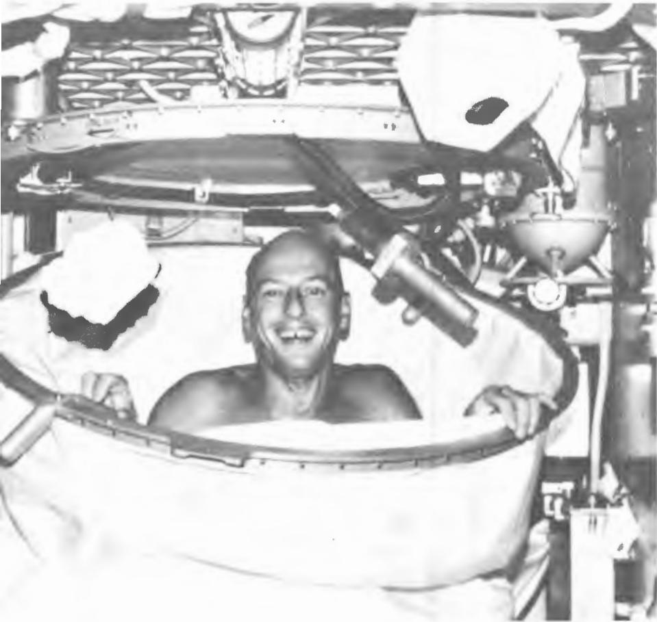
*Astronaut Charles Conrad, Jr., bathes in the shower facility in the Skylab 1/2 space station cluster. The shower curtain is pulled up from the floor and attached to the ceiling. Water flows through a push button shower head attached to a flexible hose, and is siphoned off by a vacuum system.*
