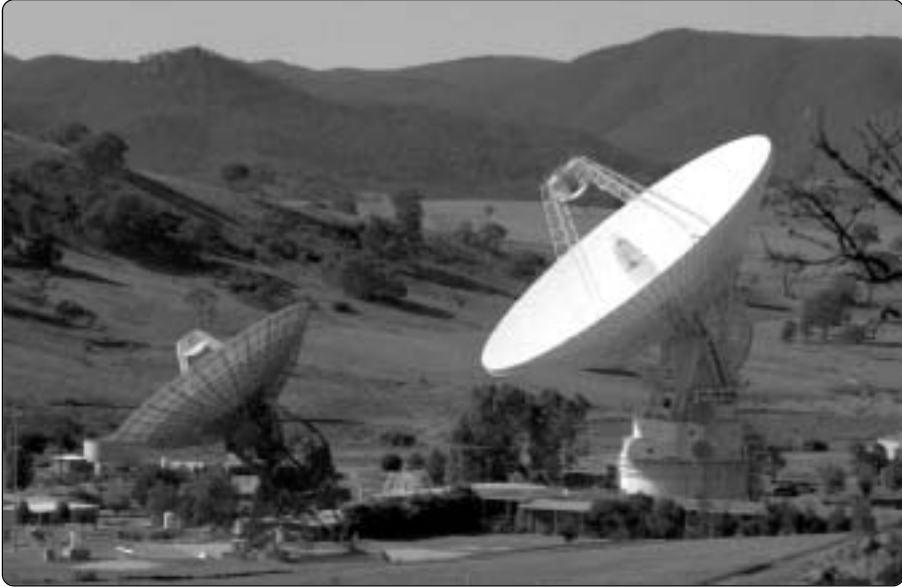
Figure 7-1. The Deep Space Communications Complex in Canberra, Australia
