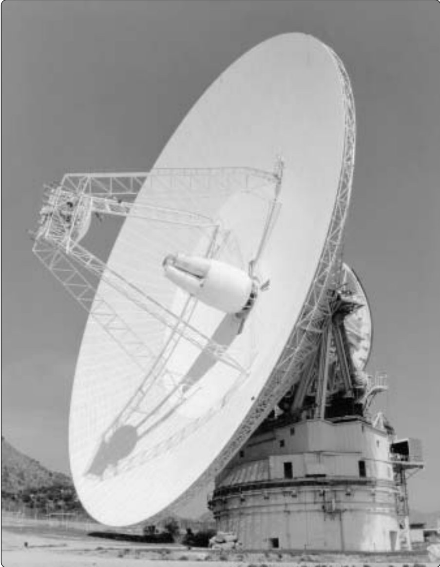
Figure 7-4. A 70-meter antenna with dual-shape reflector design.
