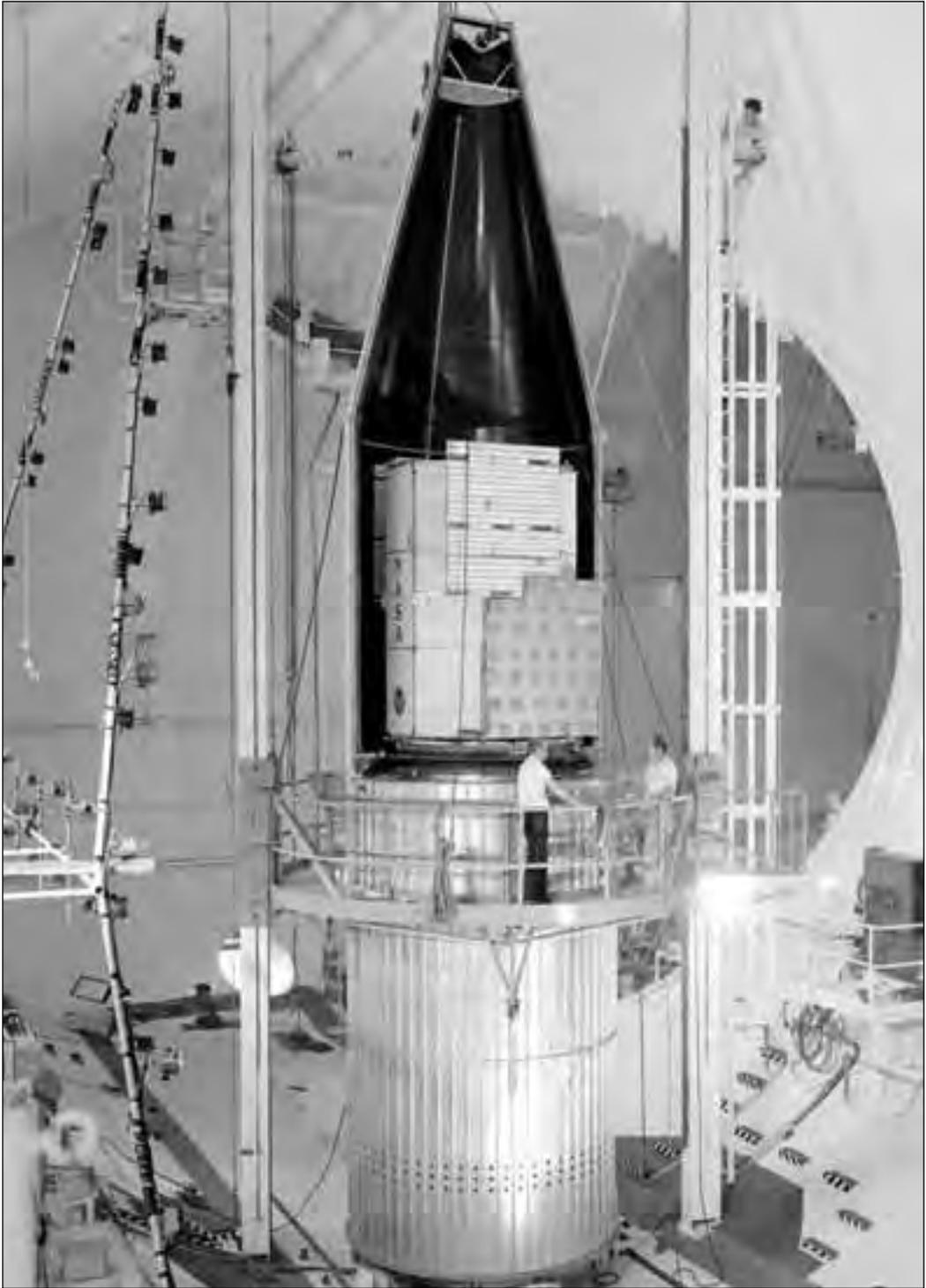
*Assembly of OAO shroud in the Space Power Facility at Plum Brook. (GRC C1965-1458)*
