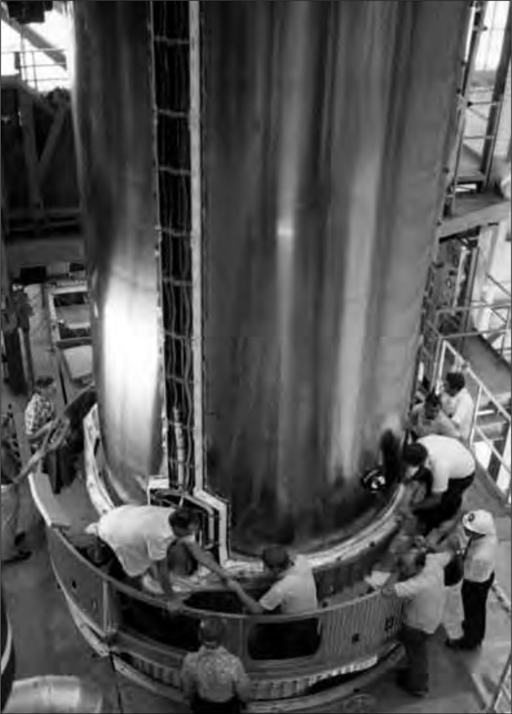
*The Centaur stage undergoes tests in the Vertical Integration Building at Kennedy Space Center on 19 October 1976. This Centaur was mated with a Titan for a Voyager launch one year later. (NASA KSC\_76PC\_0526)*
