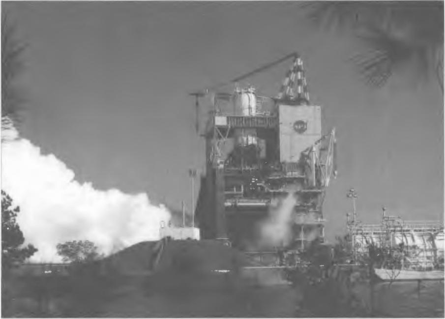
A cloud of hot steam boils out of the flame deflector at the A-1 test stand during a test firing of a Space Shuttle Main Engine in 1988 during the NASA "return-to-flight" program. (SSC-88-072-2)
