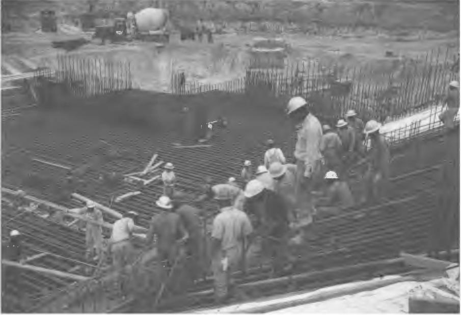
*Construction crews install steel reinforcing rods at the base of what became the A-2 test stand. The excavation for the stand went down some 50 feet with steel H-beams driven approximately 95–100 feet deeper to form a foundation for the huge piers of the test stands. (SSC-64-134C)*
