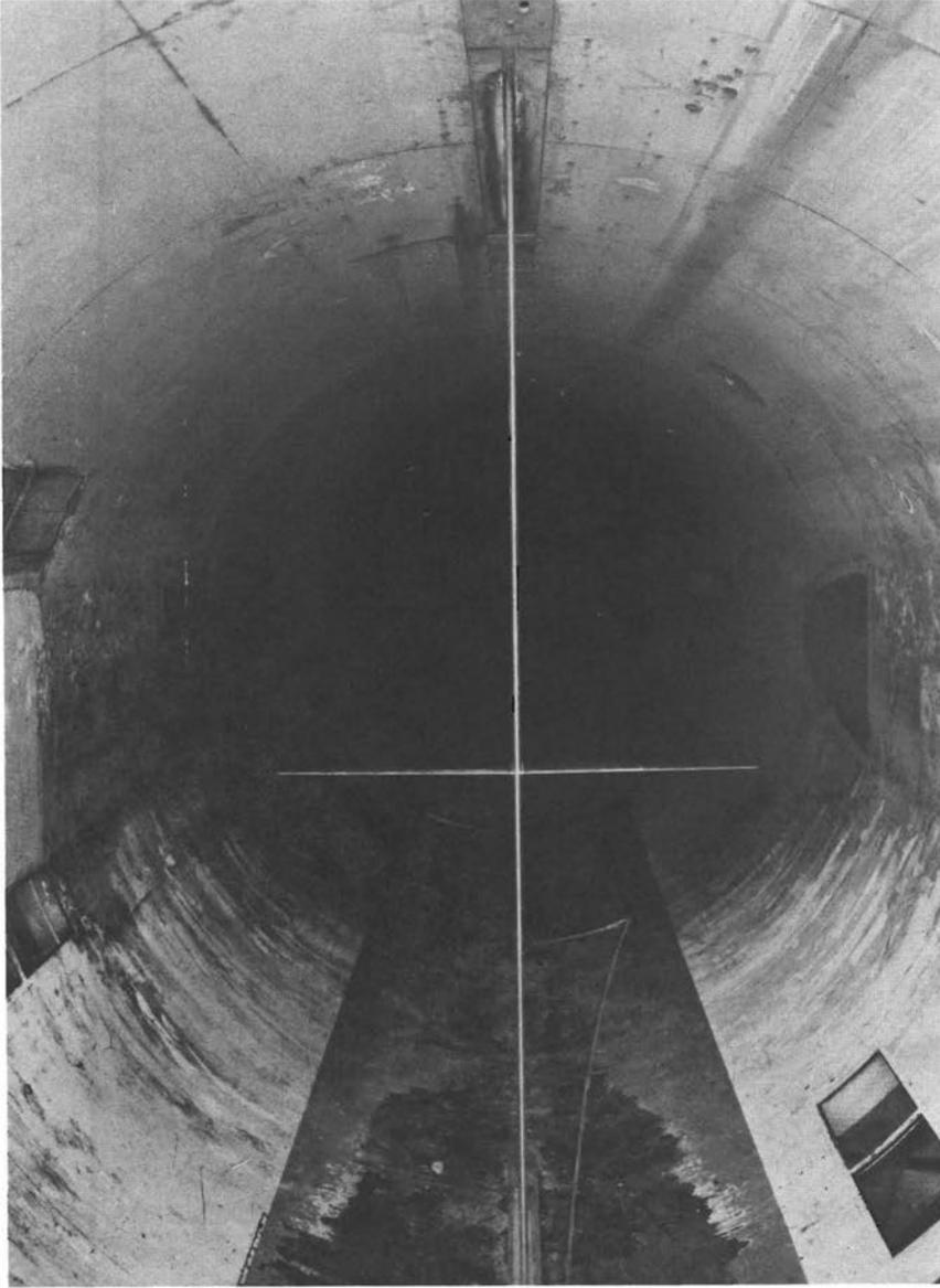
FIGURE 15.—Center-plate support for wing testing installed in the re-powered 8-Foot High-Speed Tunnel, 1945.
