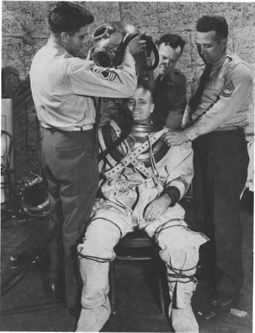
FIGURE 27.—Ray H. Wright, designer of the slotted throat, dons a diving suit for protection against noise and heat in early runs in the test chamber of the 8-foot slotted tunnel.
