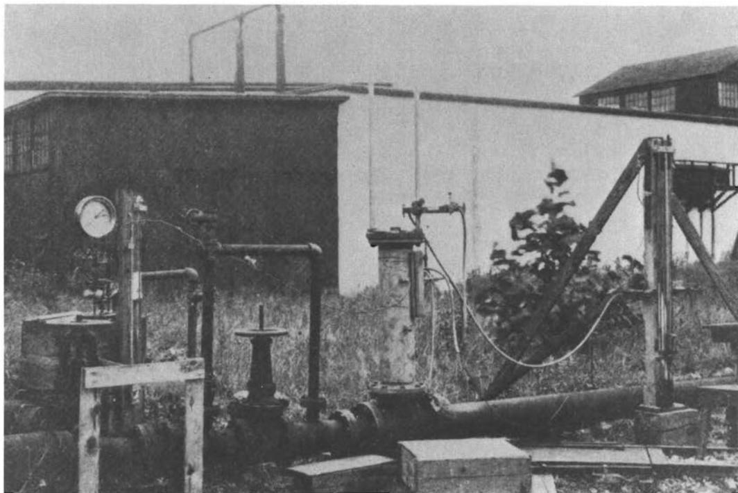
**FIGURE 10.**—*The first American facility capable of very high subsonic and low supersonic speeds, Mach 0.95 and 1.08. Briggs' and Dryden's 2-inch jet at the Edgewood Arsenal, 1926. Jet is at the top of the pipe in the center. Test airfoil is seen rotated out of the jet; single pressure tube from airfoil attaches to manometer at right.*
