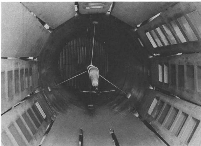
FIGURE 28.—View of the 8-foot slotted throat showing diffuser-entrance flaps.
