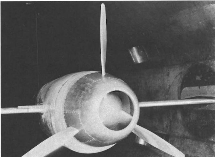
FIGURE 30.—*The 200-hp Emergency Propeller Dynamometer in the 8-Foot High-Speed Tunnel with 4-foot diameter standard blades.*
