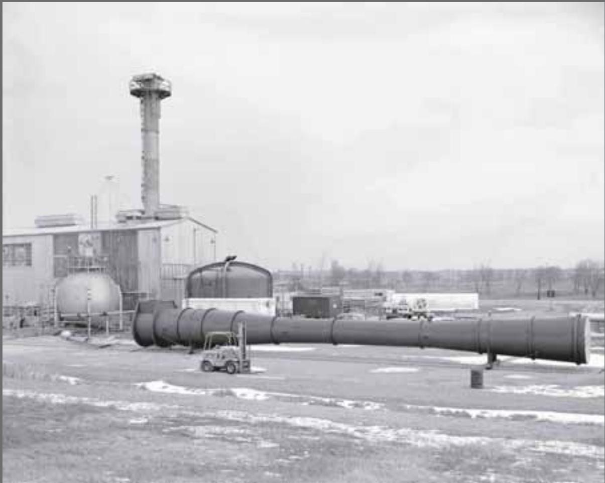
*Image 108: The Hypersonic Tunnel Facility was capable of creating air velocities and temperatures that simulated flight speeds of seven times the speed of sound, at an altitude of 120,000 feet. (1969) (NASA C-1969-00725)*
