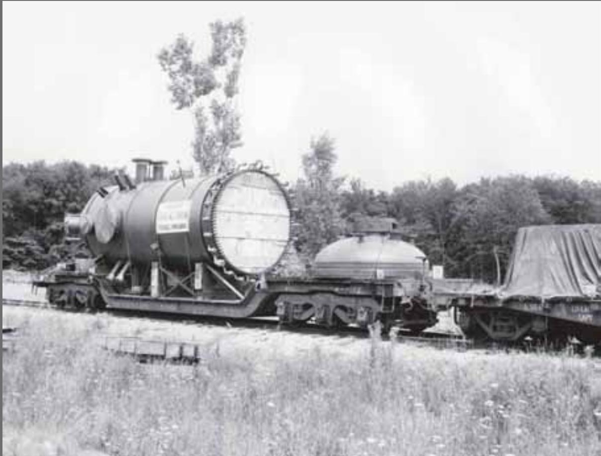
*Image 45: The pressure tank was shipped to Plum Brook via railway, and transported to the reactor facility on a flatbed truck. The tank was then rolled to a crane, which lifted it into place at the center of the unfinished quadrant area. Several pipes jutted out from the tank. These “test holes” would be used to transport experiments to the reactor core for radiation during its operating cycles. (c. 1959) (NASA C-2003-833)*
