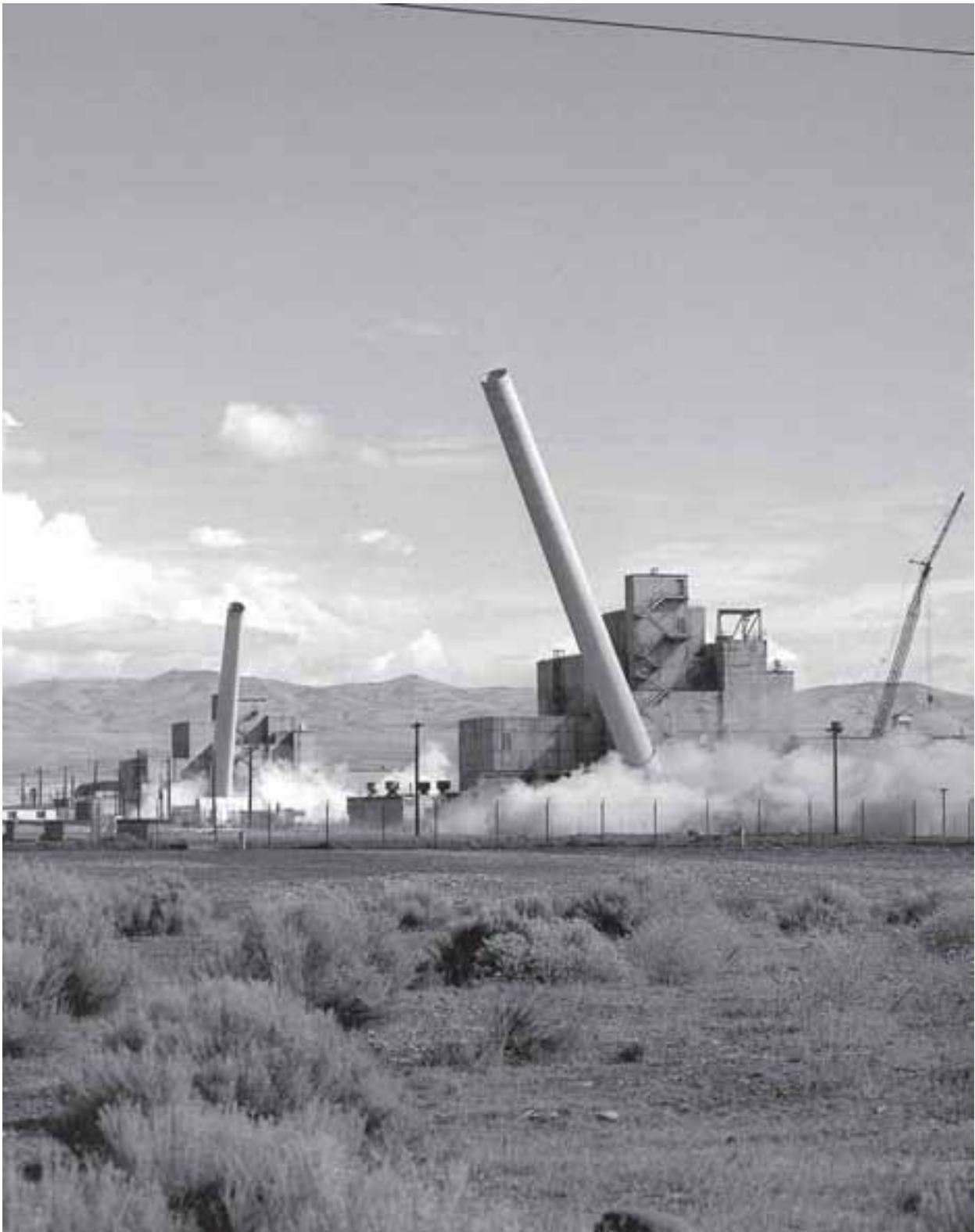
*Image 122: Two stacks are felled simultaneously during the decommissioning of the Hanford reactor. In recent years, several other reactors besides Plum Brook have been decommissioned. Successful decommissioning projects include the Watertown Arsenal, Shoreham, the Saxton Nuclear Experimental Corporation, Argonne, Pathfinder, Elk River, Fort St. Vrain, Shippingport Nuclear Power Station, and Trojan. (1977) (Department of Energy Photo 1001138)*
