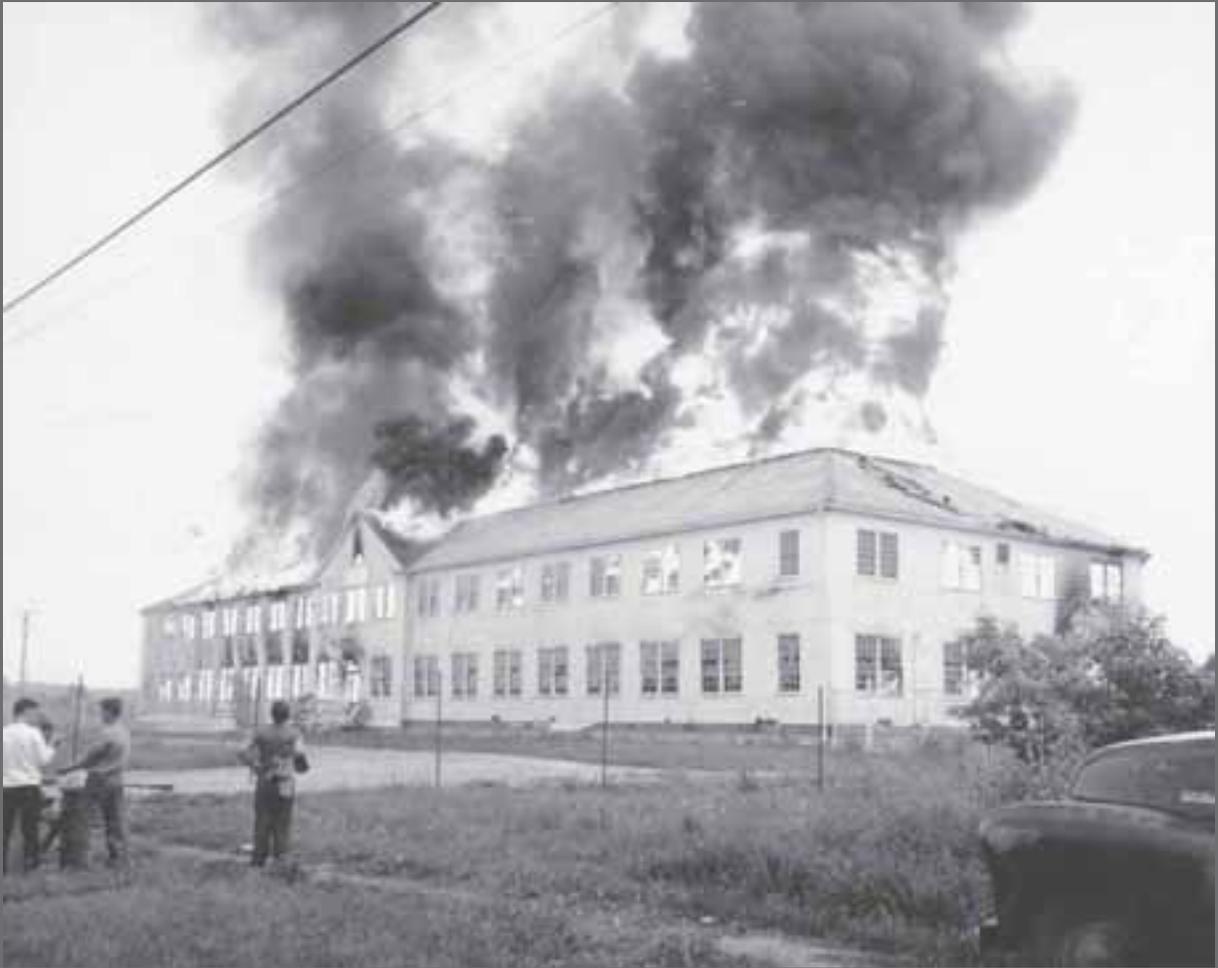
*Image 40: Controlled fire to demolish unwanted Ordnance Works structure. Upon taking possession of Plum Brook, the NACA inventoried all the Ordnance Works structures and decided to retain forty-one of them, demolishing over 600 other buildings. In addition, three TNT areas and underground waste disposal lines had to be destroyed and decontaminated. (NASA C-2003-829)*
