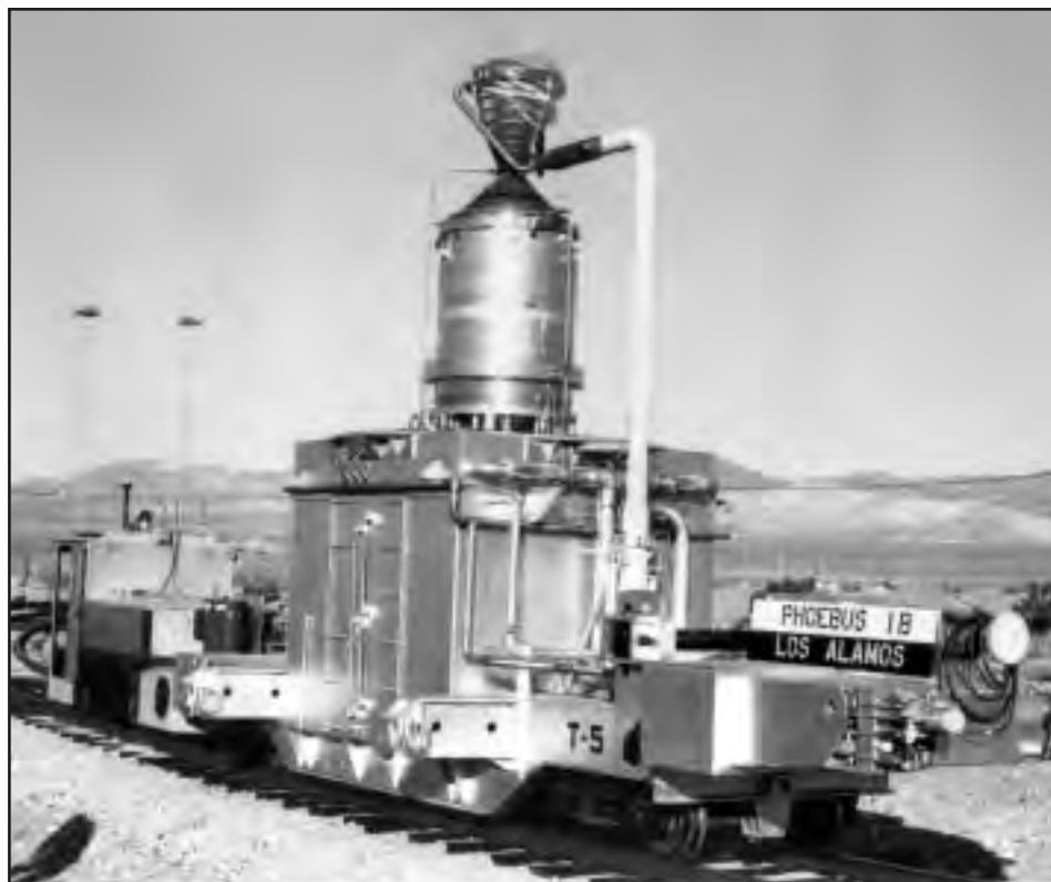
The Phobos 1B nuclear thermal rocket engine test reactor was created to further redefine the engineering aspects of a nuclear propulsion system. This particular unit was successfully tested in 1967.
