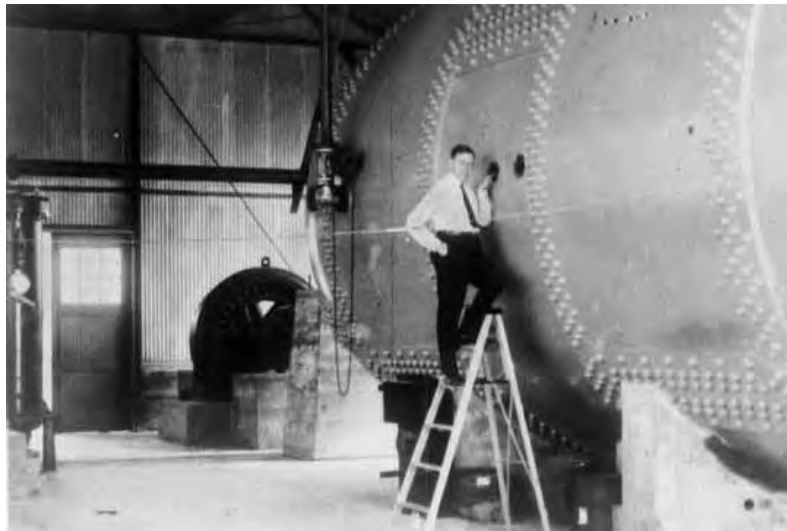
Figure 9. Dr. Max Munk, the famed inventor of the VDT concept, inspects the tank after it was mounted on concrete pads in Building 582. Dr. Munk has turned toward the front of the building facing the Back River. The photograph was probably taken in the summer of 1922, but the specific date indicated (6/1/1922) is questionable.
