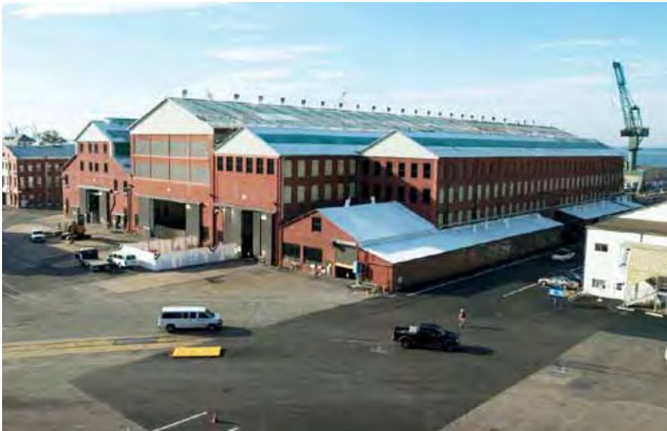
Figure 3. View of the massive 120-year-old machine shop buildings at Northrop Grumman Shipbuilding in Newport News. (Photo courtesy of Northrop Grumman Shipbuilding, Newport News)
